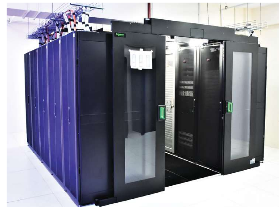
Figure 3: NESCO data center server room.
