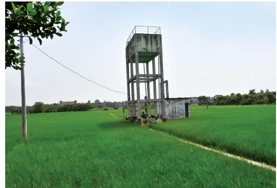
Electricity distribution to irrigation customer in Hatibandha upazilla under Sales & Distribution, NESCO PIC, Hatibandha, Lalmonirhat.
