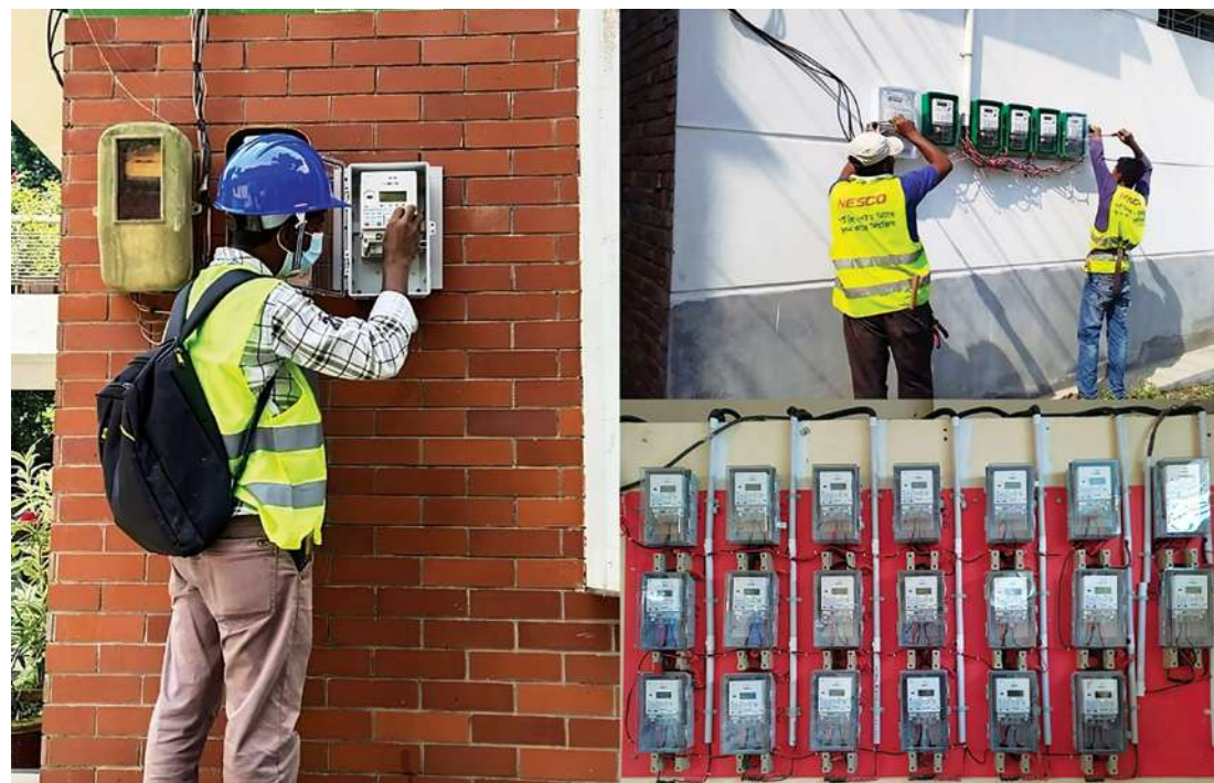
Installation of Smart Meter in Rangpur under "Smart Meter Installation Project in NESCO Area of Rajshahi and Rangpur Division".
