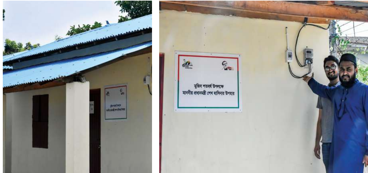
Electricity connection provided by NESCO to The Ashrayan Project under Sales and Distribution Division, Kashiadanga, NESCO PLC.
